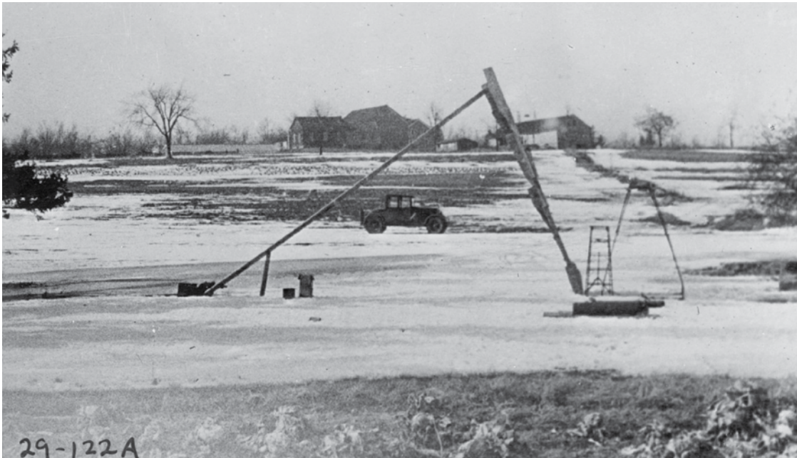
◀ This photo is believed to show the testing apparatus for Robert Goddard's historic March 1926 launch of the first liquid-fueled rocket. Esther Goddard recorded the test on her 16 mm film camera and extracted this still, captioning it "testing frame and wind break" in the album "The Goddard Rocket Researches: A Photographic Record."
