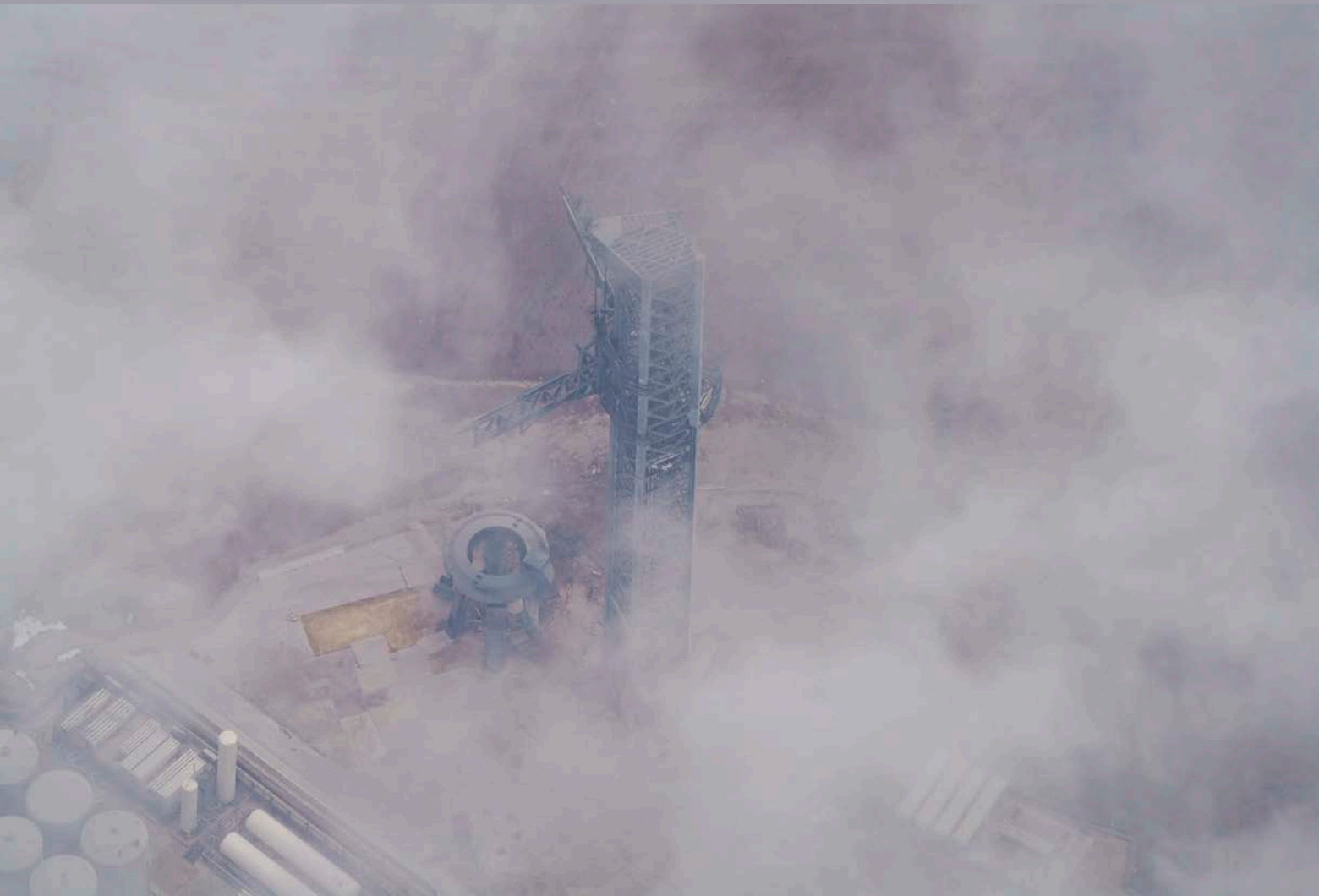
AFTER Chunks of the concrete launch pad were blown away, exposing the ground beneath, as seen in this drone photo. RGV Aerial Photography
